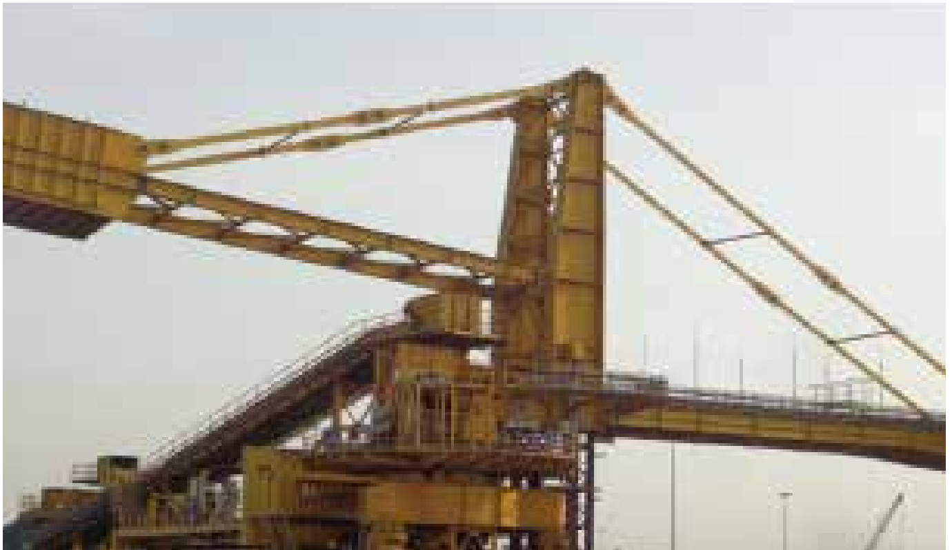
Stacker Reclaimers - Erected at Jharsuguda, Odisha, India
