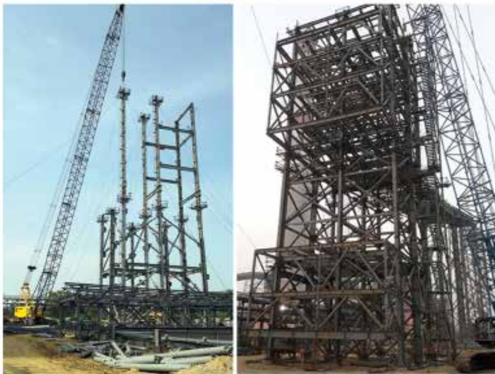
Fabrication and Erection of High Elevated Structurals
